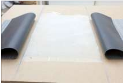
Picture 5: How to start installation of the rolls
