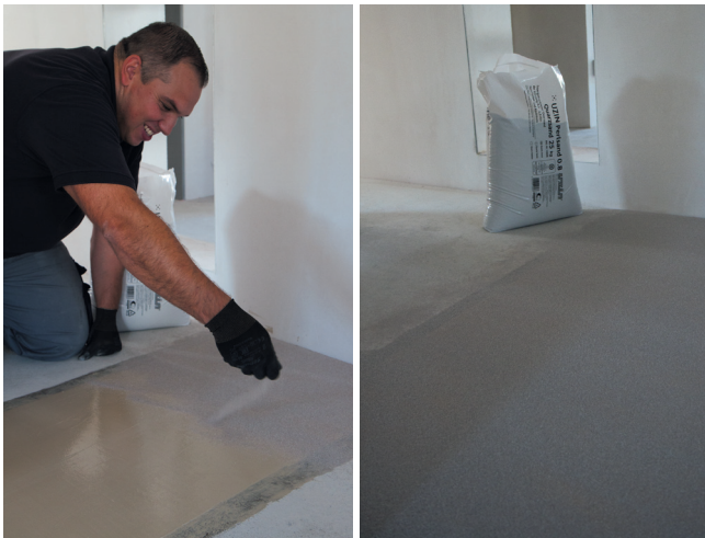
Sand UZIN MK 92 S with UZIN Fine Sand 0.8 for subsequent levelling work.
